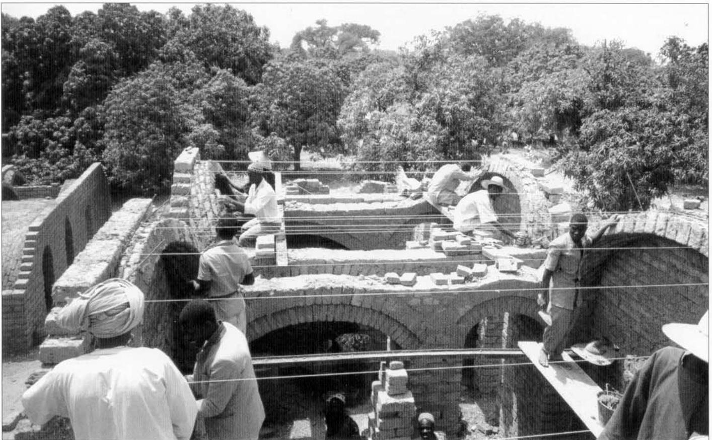
Figure 2 “Alcove” building under construction. Note the use of strings as a guide, the practice of starting the vault from both ends simultaneously, the use of off-centred vaults and open arches to create a spacious interior.
