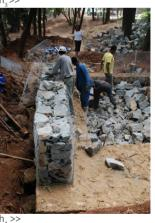
f >> 'foundation' section g >> final floor plan  $h_1 >>$  preparation of stone blocks  $h_2 >> 1^{st}$  layer of stones  $h_3 >>$  stone-mud mortar base  $h_4 >>$  filling out gabions with stones.
