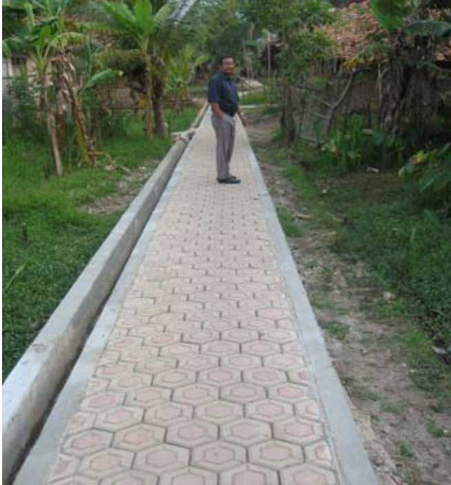
A newly constructed footpath in a community in Serang, West Java
