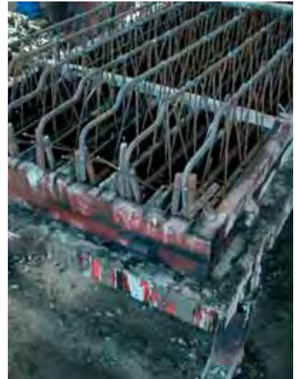
The mould with the reinforcement ready for casting
