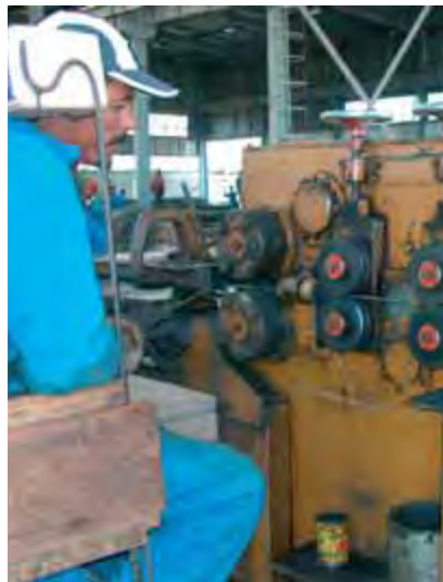
Stretching of reinforcement
