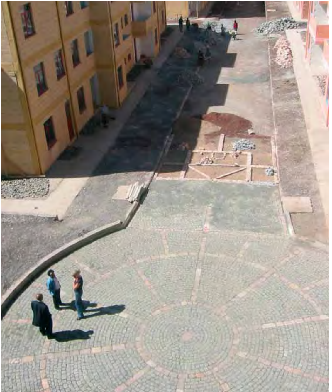
Stonework for Bole Gerji site
