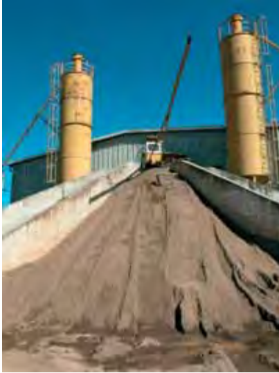
Large scale storage of mineral aggregates
