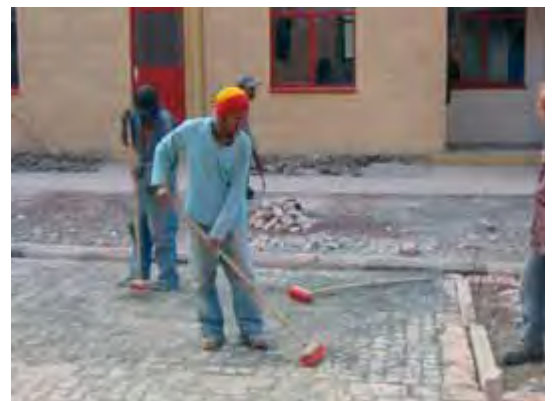
Flushing of gaps
