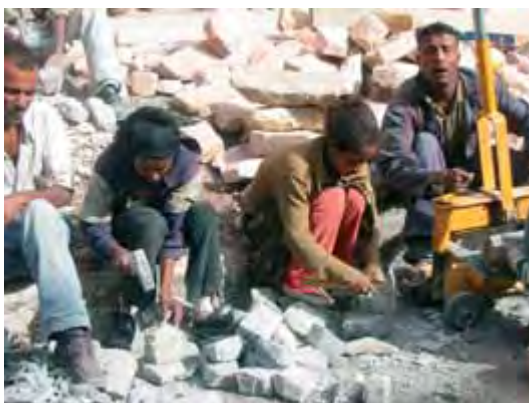
Provision of hand hewn stones for the pavement
