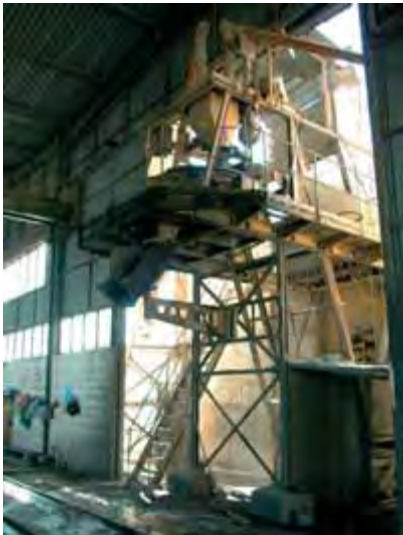
Large scale concrete mixer
