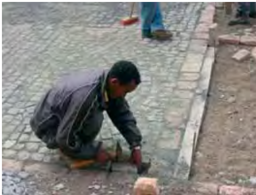
Paving of complex stone patterns
