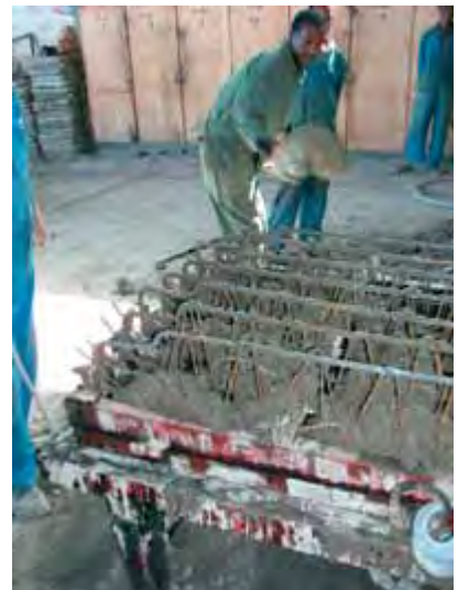
Casting of concrete into the mould mounted on a vibrating table
