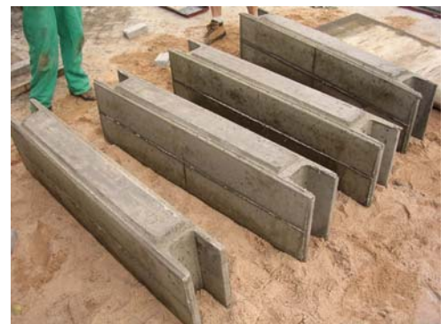
37 | Final result after casting and demoulding
