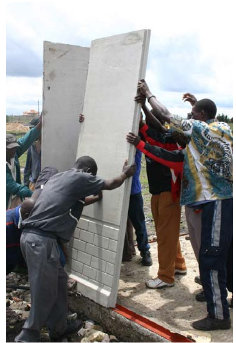
7 | Erection of an Eco-home
