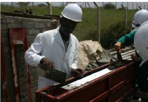
36 | Casting of the elements
