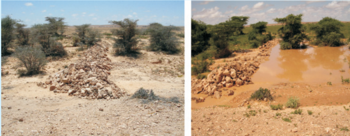
Simple rock dam at Awsane built in March 2005 (left) before the rains and two months later after rain (right)
