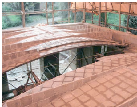
h >> Unreinforced timber vaulted floor system of the SUDU housing prototype: a) simple, single-curved barrel vault with stiffening diaphragms, to be stabilized with a pumice/lime fill.
