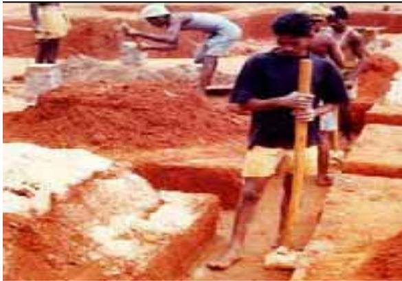
Fig 2: rammed earth foundation
