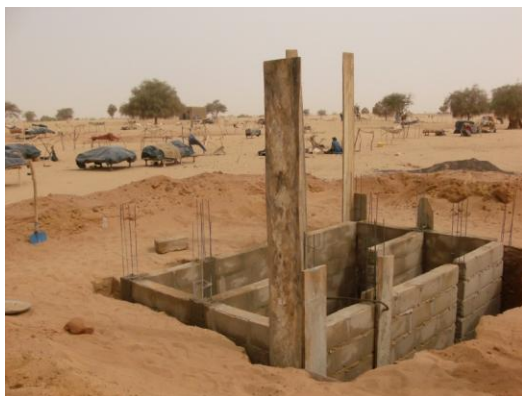
Latrine and shower blocks are under construction.
