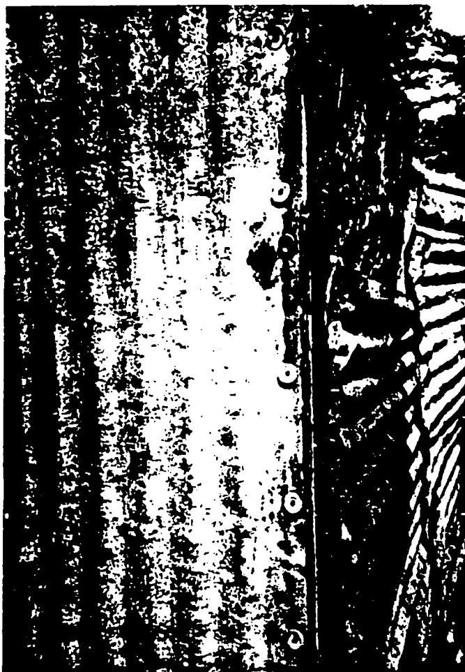
Figure 6: Local creativity in Anivorano – use of metal bottle caps as washers for roofing nails.
