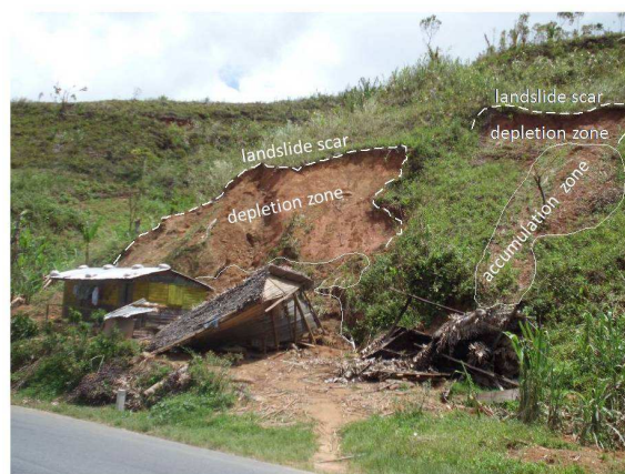
Figure 8: Destruction of house due to translational landslide (PK 189 of the RN2)
