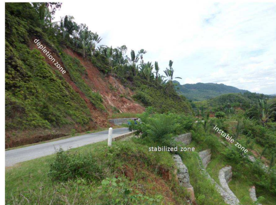
Figure 11: Technical measurements of stabilization (PK 95.200 of the RN25)
