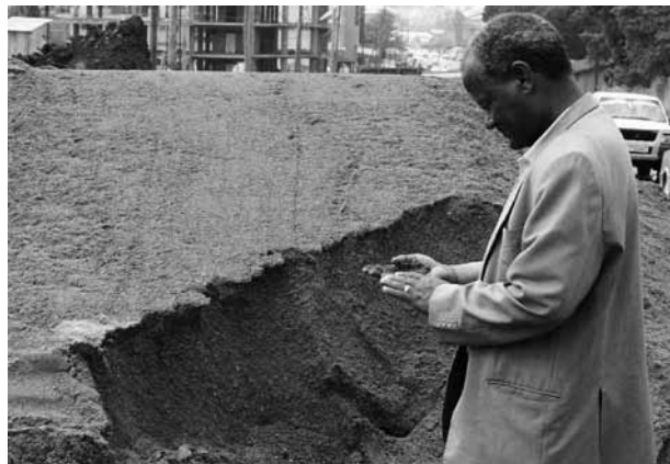
Figure 27: Quality checks on building materials are crucial to ensure a high-quality result. Lideta, Addis Ababa. © UN-HABITAT/ Katherine Hegab
