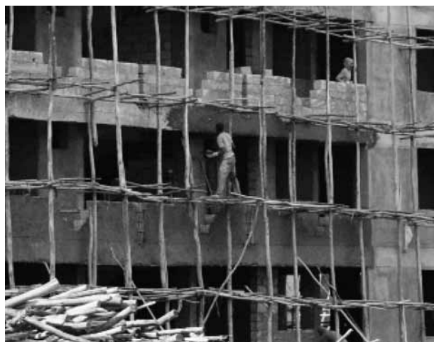
Figure 28: Workman applying plaster to the first-storey of a condominium block. Bole Summit, Addis Ababa. © UN-HABITAT/ Katherine Hegab
