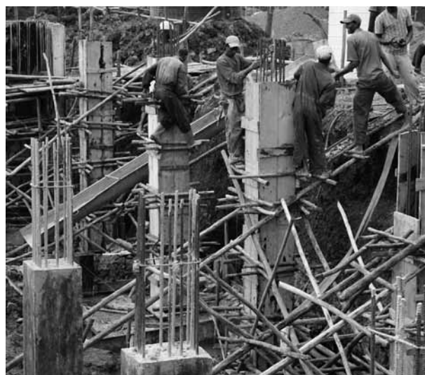
Figure 31: Labourers building the foundations for Lideta condominiums Lideta, Addis Ababa.
