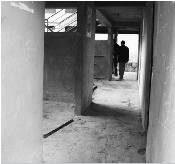
Figure 35: Significant improvement could be made to the design of the built environment to improve the responsiveness to occupant needs and lifestyles.
