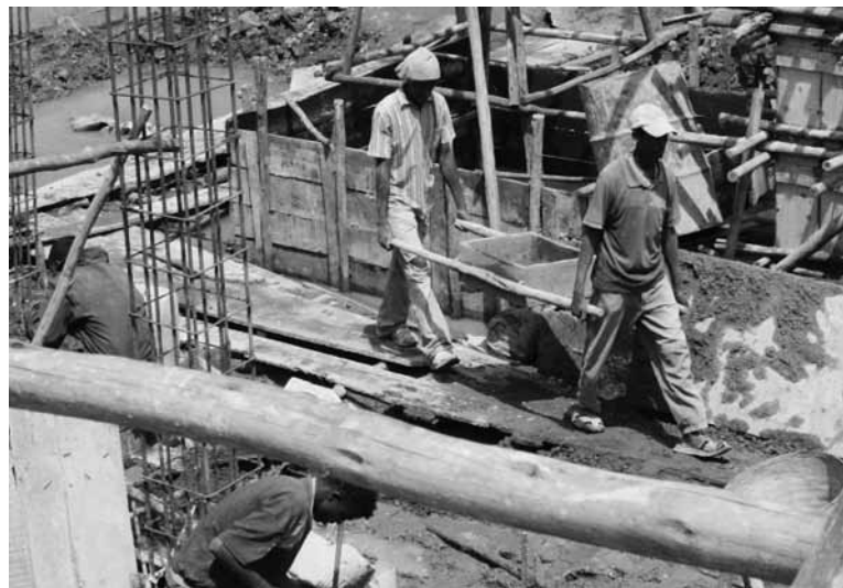
Figure 26: Construction of Bole Summit, Addis Ababa. © UN-HABITAT/ Katherine Hegab
