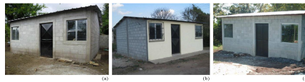
Figure 1. General view of a single house of this building type. a) Quiché (Northwest of Guatemala) [3], b) Chimaltenango (Center of Guatemala) [4], c) Alta Verapaz (North of Guatemala) [5].
