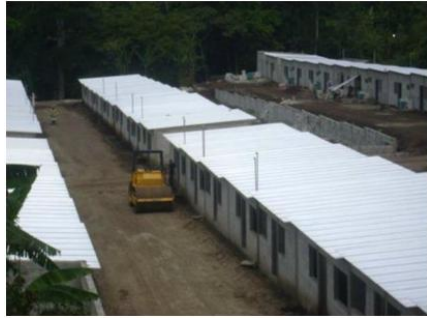
Figure 2. View of several buildings with adjacent walls to neighboring buildings [6].
