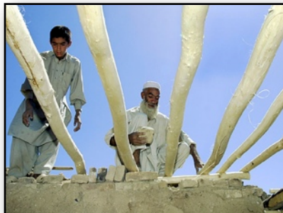
Reconstruction begins after an earthquake.
