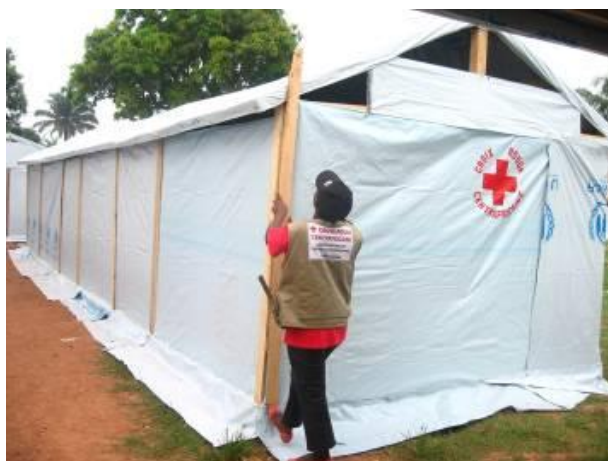
CAR Red Cross volunteers constructed shelters for flood-affected persons/Yvette Mve/International Federation
