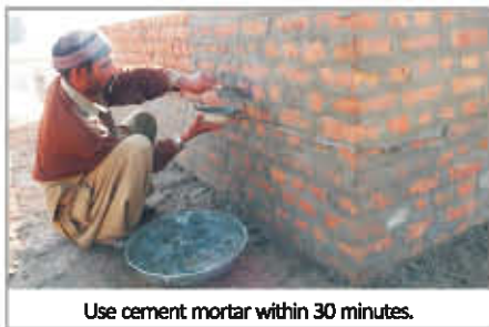
Use cement mortar within 30 minutes.
