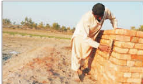
Use steel brush to remove mud/dust from the joints.
