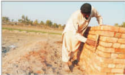
Use steel brush to remove mud/dust from the joints.
