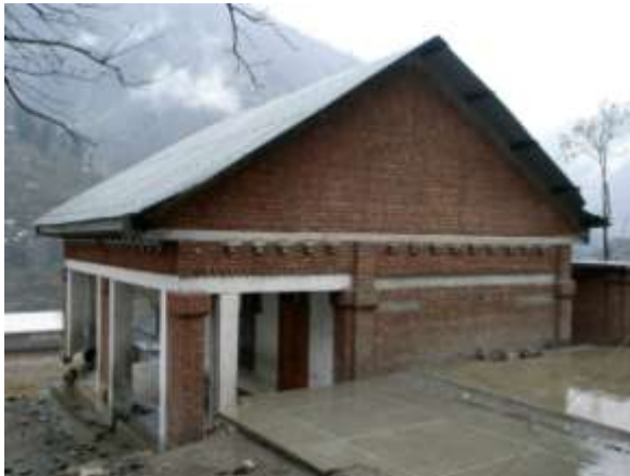
Above: A pre-earthquake school building in Pakistan incorporating seismic mitigation measures. Current regulation in the country would prohibit the unrestrained gable end. Nevertheless the building survived with very little damage and remains in use today.
