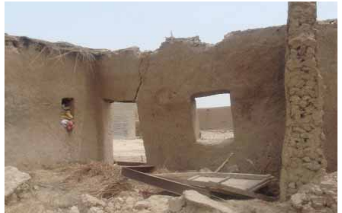
Balochistan Mud lumps shape of balls are stacked to make mud wall.
