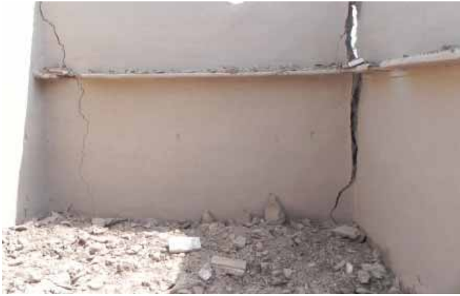
Sindh Corner failure due to settlement of foundation.
