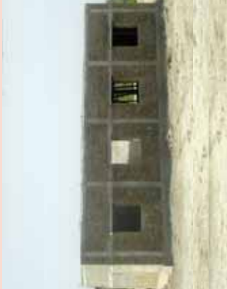
P4 RC Confined brick masonry Size 1 Room (15X15 ft) Cost=PKR 200,000
