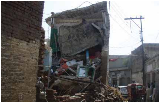
Collapse of wall causing RC roof to collapse.
