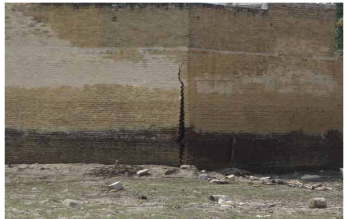
KP Poor corner brick masonry.
