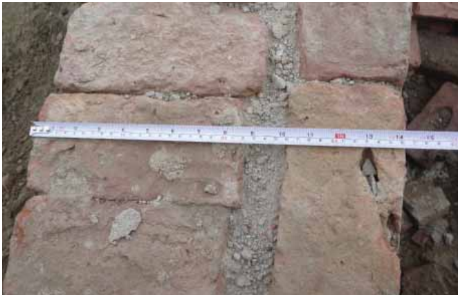
More than one inch wide joint filled with mud mortar.
