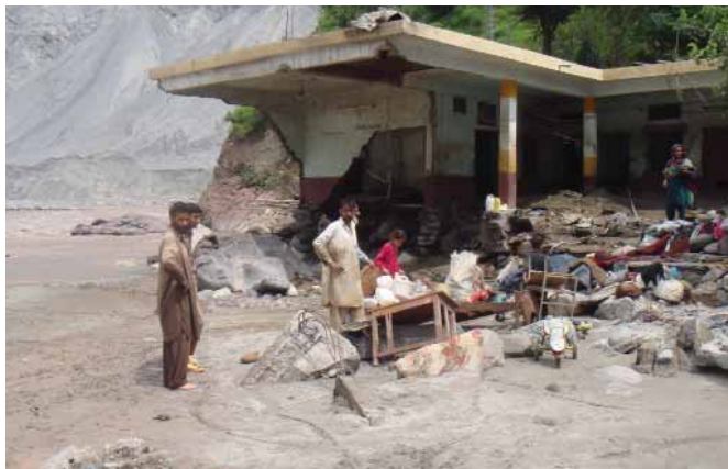
AJK Portion of the home washed away and foundation is eroded.
