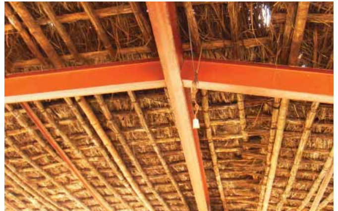
Punjab Roof made with girders, bamboo and kana.
