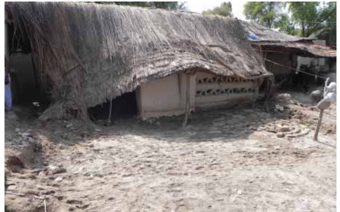
Sindh Collapse of walls due to standing water.
