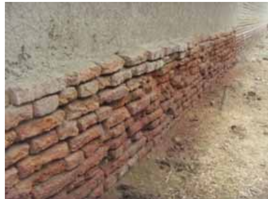
Bricks deteriorated due to seepage
