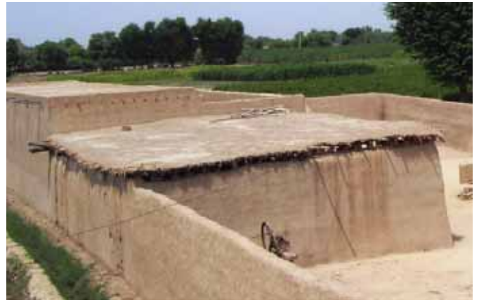
Sind Flat mud roof with timber, patar and mud.
