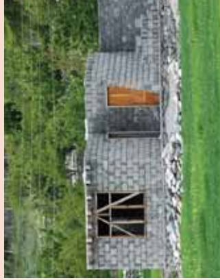
P3 Unreinforced block masonry C/S Mortar Size 1 Room (15X15 ft) Cost=PKR 160,000
