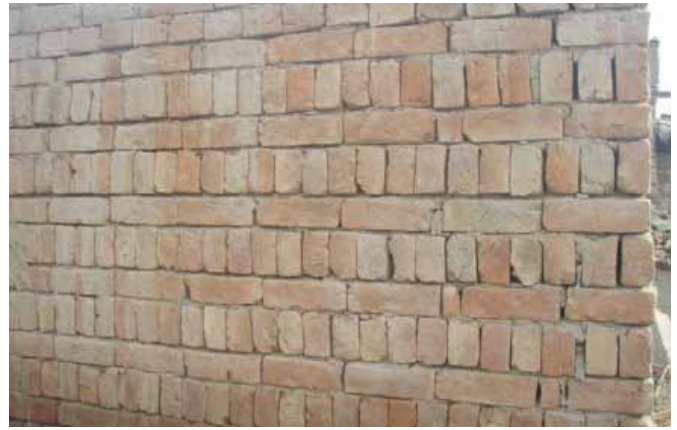
Bricks are placed vertically in alternate courses.
