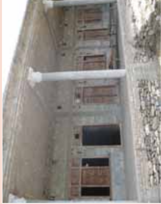
P5 RC Confined block masonry Size 1 Room (15X15 ft) Cost=PKR 200,000
