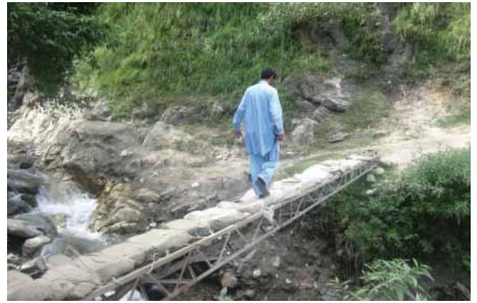
Temporary access bridge using salvage material.
