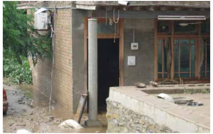
KP Column and girders do not have anchorage.
