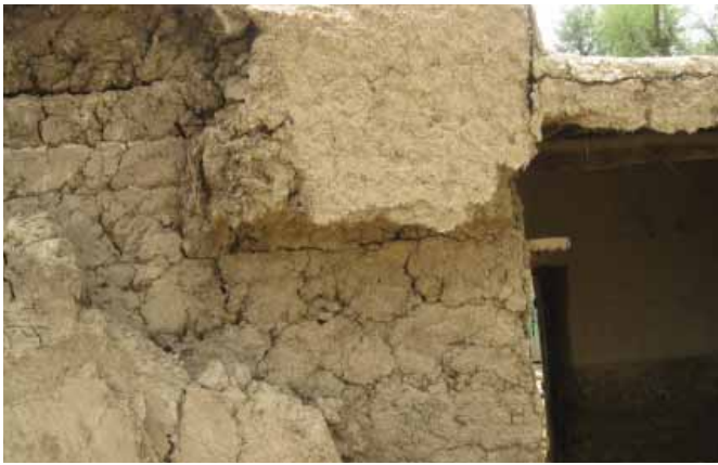
KP Delamination in mud.
