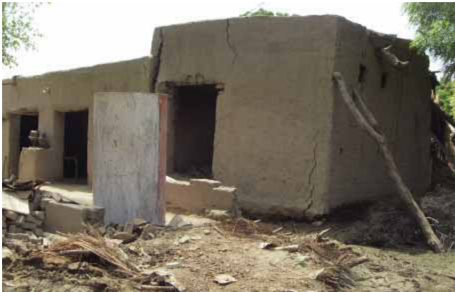
Sindh Foundation soil got moist due to standing water around it causing settlement of foundation.
