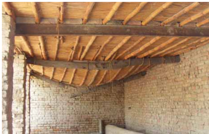
Sagging of roof caused by prolonged rains, as mud gets saturated and load increases.
