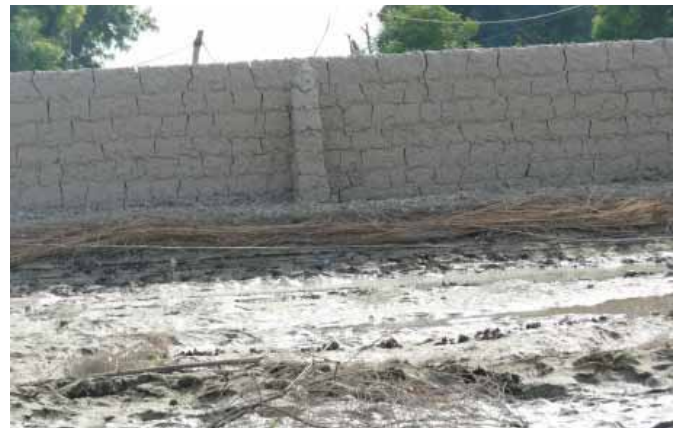
Use of buttressing in boundary wall.
