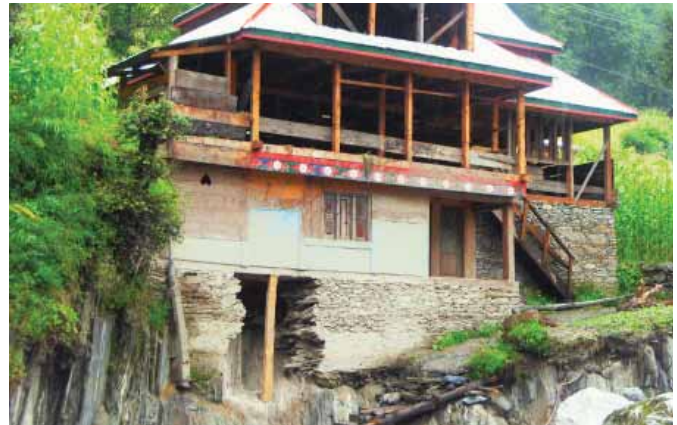
Stone masonry front wall fell down.
