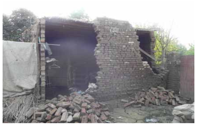
KP 4.5 inch thick wall of brick masonry in mud mortar.
