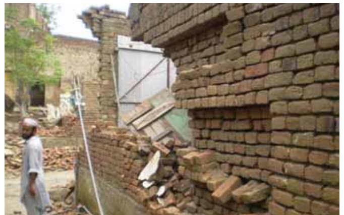
KP Delamination in brick masonry.
