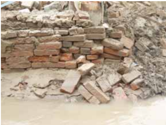
Bricks absorbed too much water and broken:
