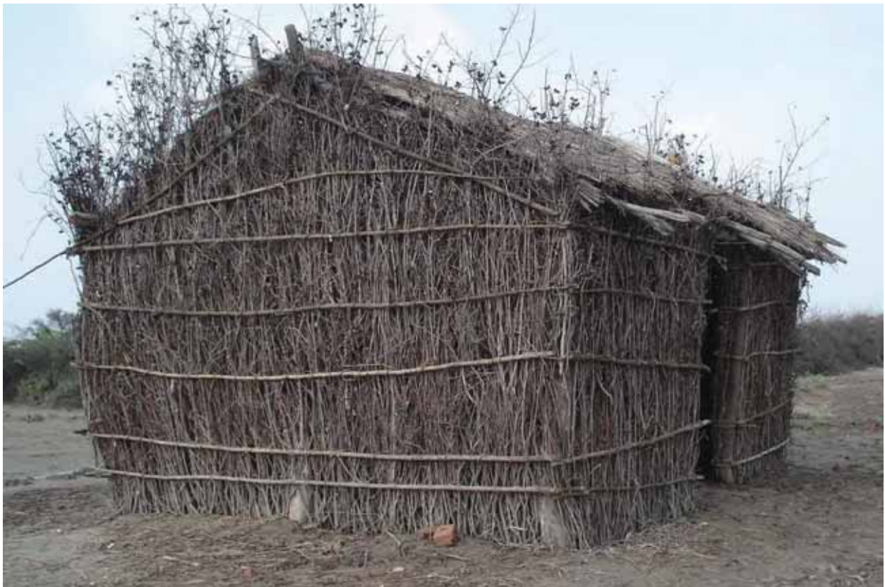
Grass house Sindh. Local grasses and reeds affected by flooding. May be improved by fixing to ground and bracing for cyclones. Household needs sanitation solutions.
