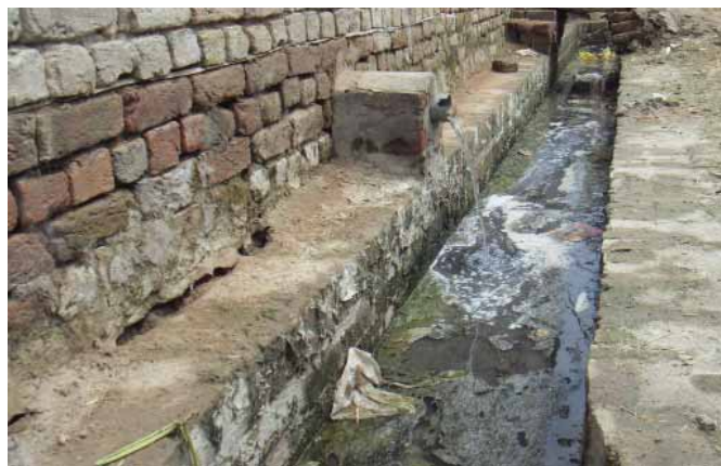
Water from washrooms and kitchens flows into streets due to the blockage of drains.
