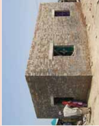
P2 Unreinforced brick masonry C/S mortar Size 1 Room (15X15 ft) Cost=PKR 160,000
