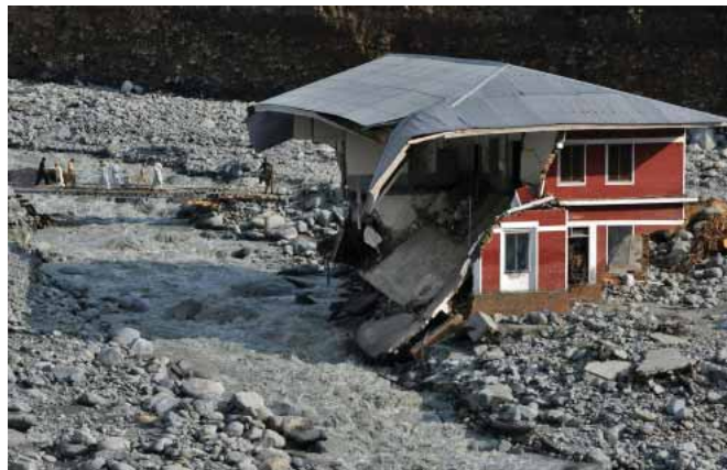
KP Due to flooding in the Nallah, building received considerable damage.
