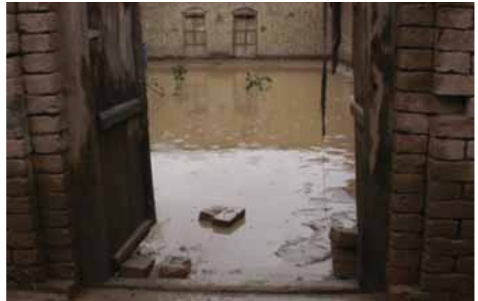
Natural ground level and finish floor level are same.
