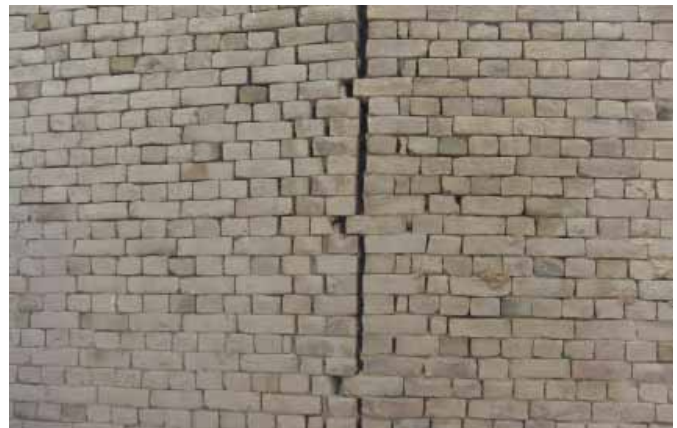
Poor interlocking between two walls.
