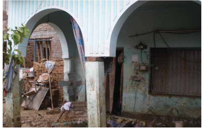
KP No reinforcement to connect arch and column.
