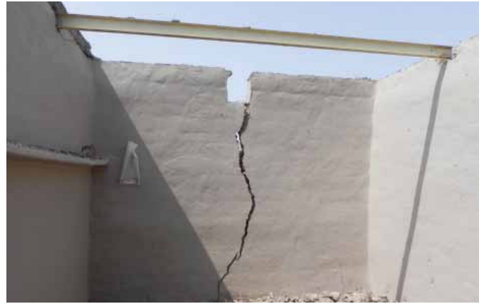
Sindh Major crack due to settlement of foundation.
