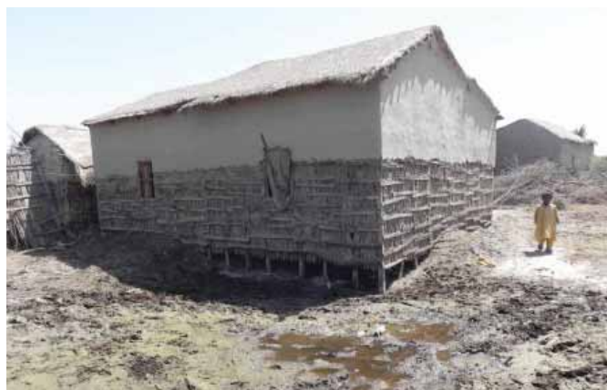
Sindh Foundation have been scoured but building is intact.
