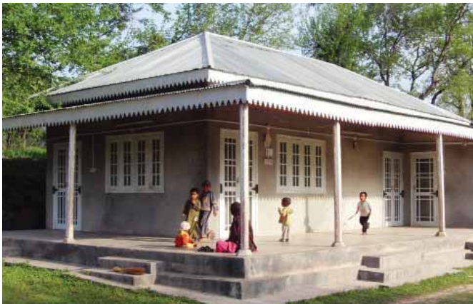
AJK Corrugated galvanized iron sheet with timber.
