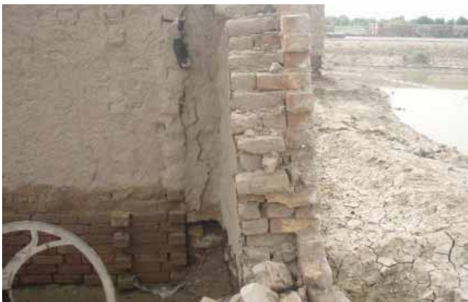
Use of fired brick on front side of wall, brick are interlocked after 5th layer.
