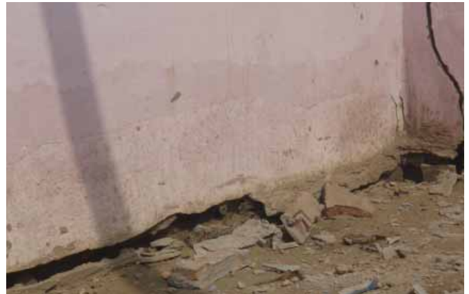
Punjab Erosion of base of wall.
