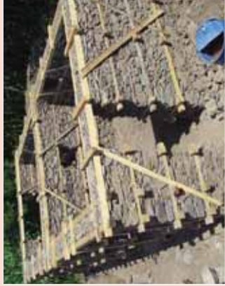
P6 Bhatar/Timber reinforced masonry Size 1 Room (15X15 ft) Cost=PKR 140,000
