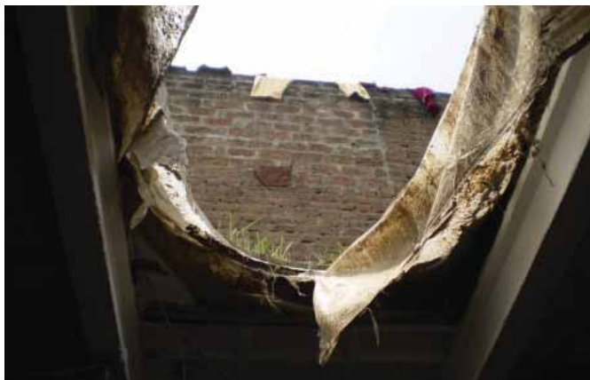
Damage to the roof made with precast concrete slab caused by extra load.
