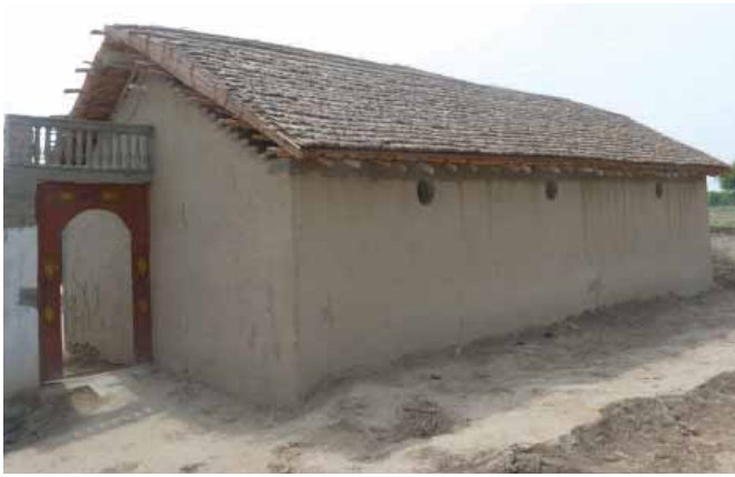
Sind Sloping Katcha roof, with bamboo and pun.
