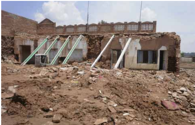
KP Girder are placed directly on wall and not anchored.
