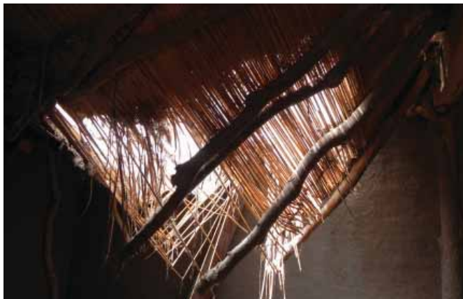
Roof failure due to heavy and prolonged rain.
