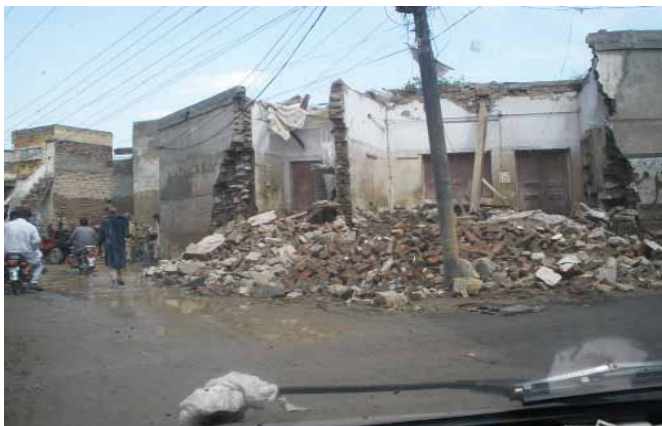
KP No connection between cross wall and long wall.
