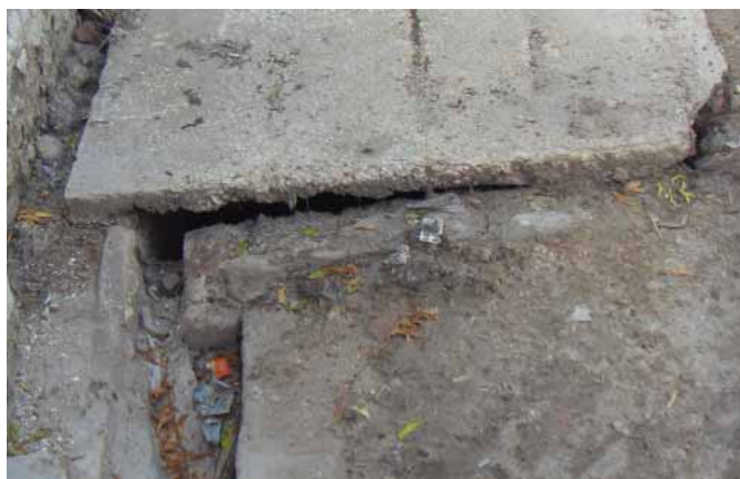
Drains are blocked by debris causing stagnation of water in streets.
