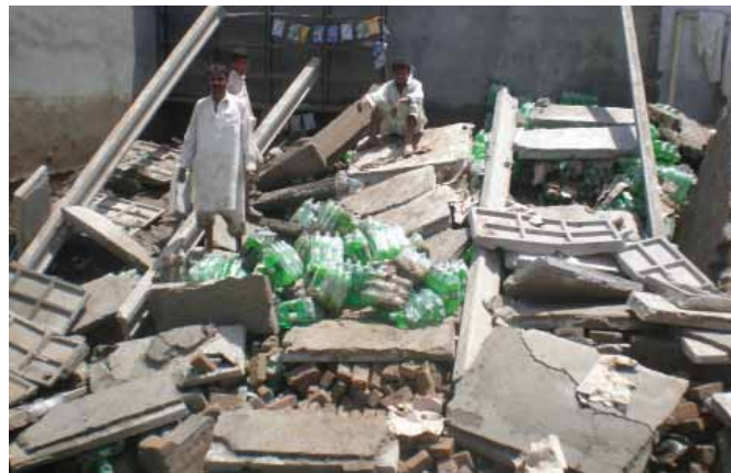
Complete collapse of roof due to heavy rain.
