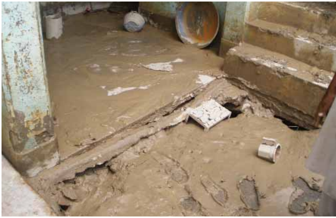
Water enters into the foundation and weaken the structure.
