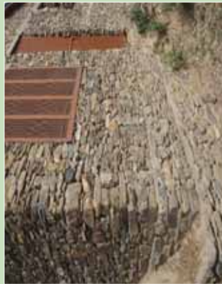
K5 Fired brick with mud mortar Size 1 Room (18X14 ft) Cost=PKR 130,000
