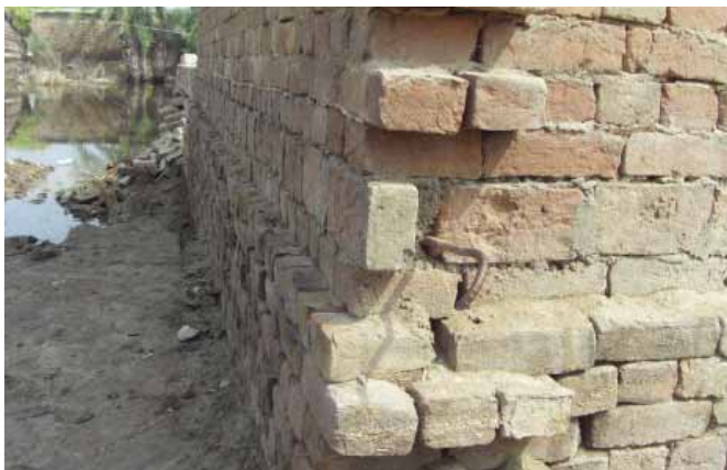
Brick reinforced beam with poor reinforcement detect.
