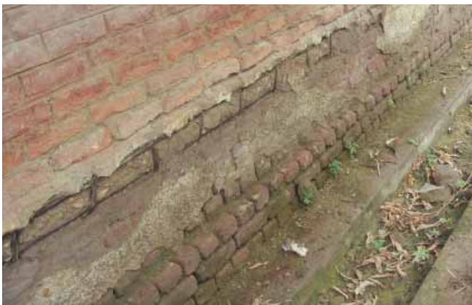
Spalling off concrete from plinth beam.
