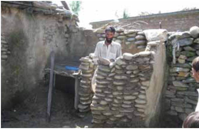
KP River stones are being used to make stone masonry in mud mortar.
