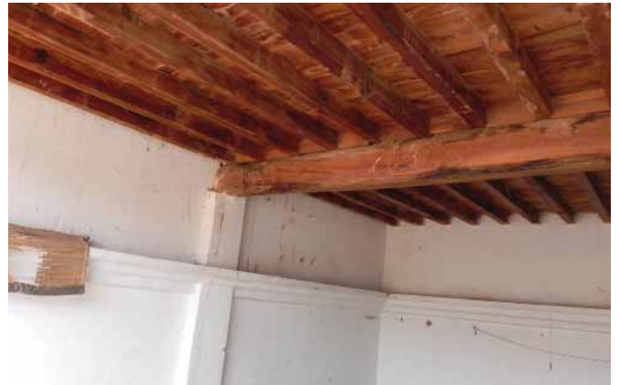
Punjab Roof with wooden beams, wooden joists and mush.
