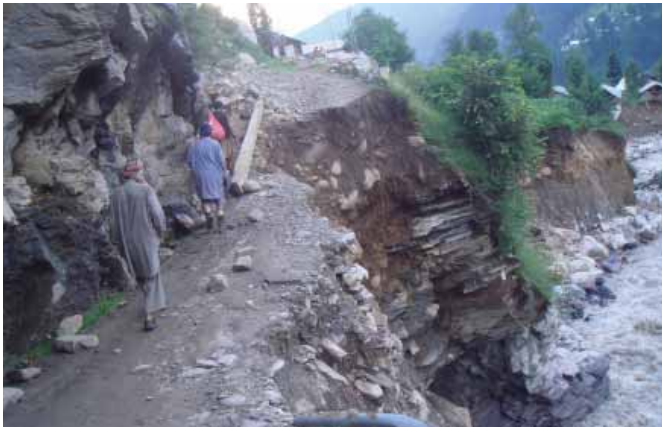
Destroyed access road caused by the landslide.
