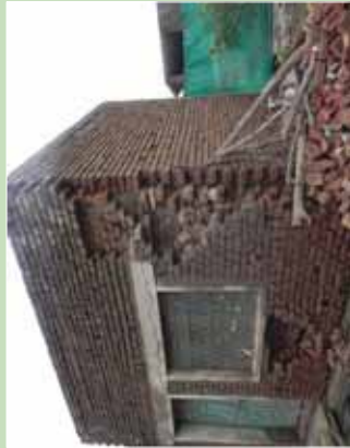
K5 Fired brick with mud mortar Size 1 Room (18X14 ft) Cost=PKR 130,000
