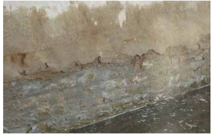
Cement mortar pointing on brick masonry in mud mortar on lower part of mud wall.
