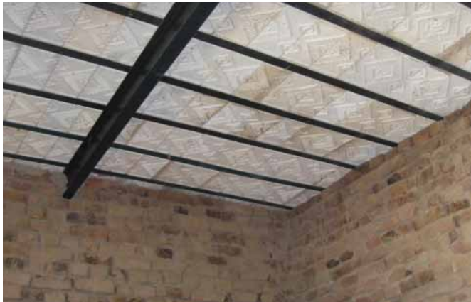
Punjab Steel girder and T-iron with brick tile roof.
