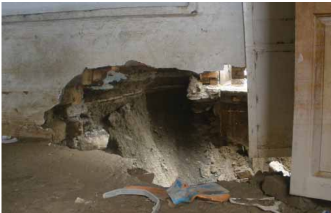
Loose fill fell down with the collapse of front plinth wall.
