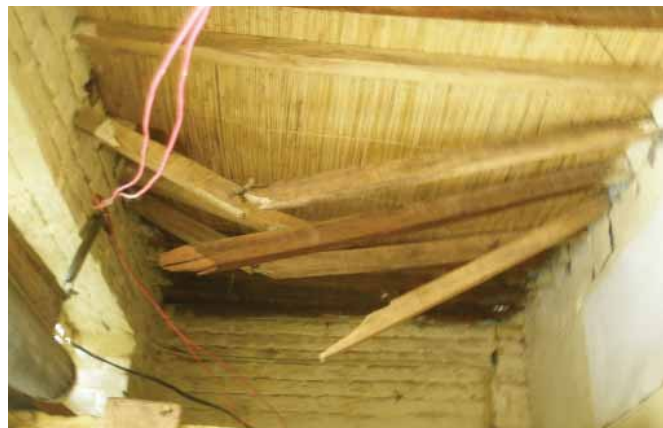
Timber beams broken due to increase load.
