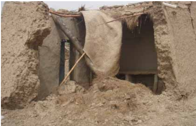
Balochistan Collapse of walls due to rain splashes.
