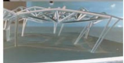
This structure makes use of both the natural compression & tension characteristics of bamboo, to explore the potential of this versatile material. The modern elements of the structure is provided by the steel connection details as well as the overall dynamic form.
