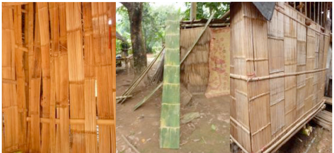
FLATTENED BAMBOO SHEETING WALLS
