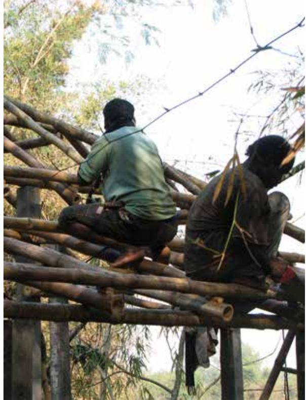
Step 2.E: tertiary roof structure attached
