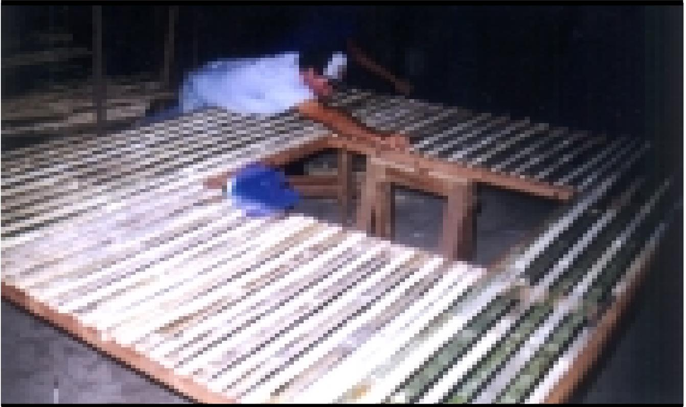
**Fig. 19:** *Panels being prefabricated for mass housing*
