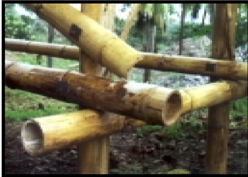
**Fig. 64:** *A joint in Group 5, with steel bolts*
