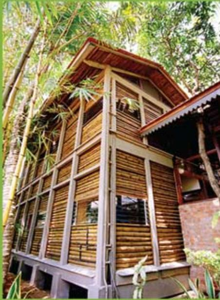
We were able to reduce the use of 70 to 80% cement and steel, by the use of bamboo, if we are to compare with a building of same design built with conventional materials.
