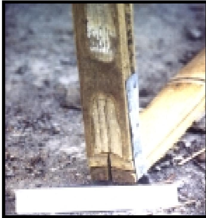
**Fig. 69:** *Joint for the lower corner of doorframes*
