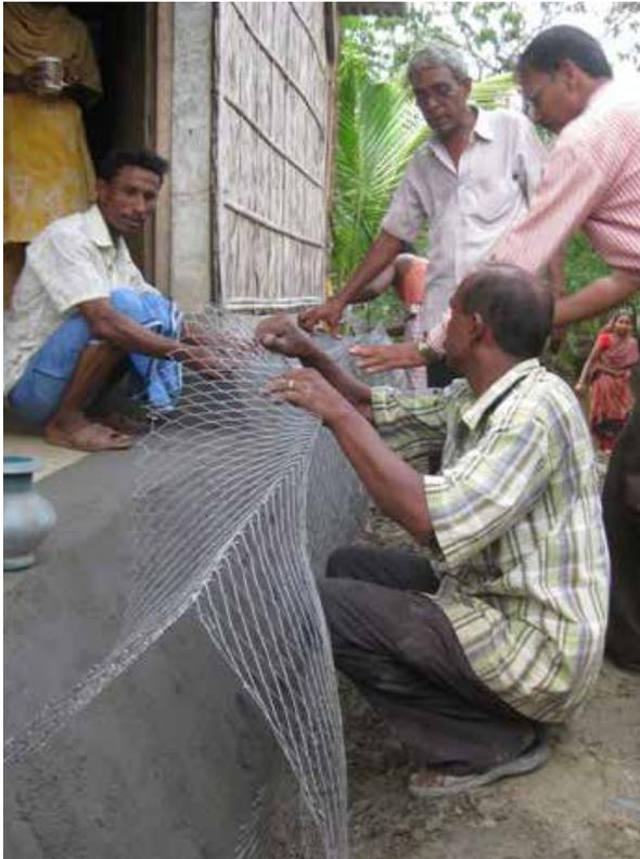
Step 3.C: erosion-prevention technique applied to exterior surfaces and slopes of plinth
