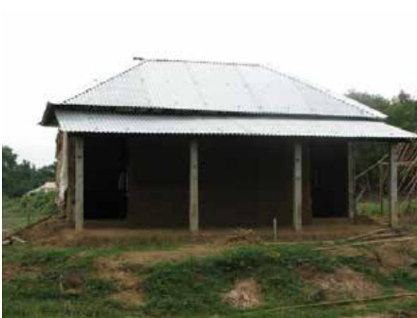
Step 4.C: ridge covers attached to CGI sheets roof structure at ridge and diagonals
