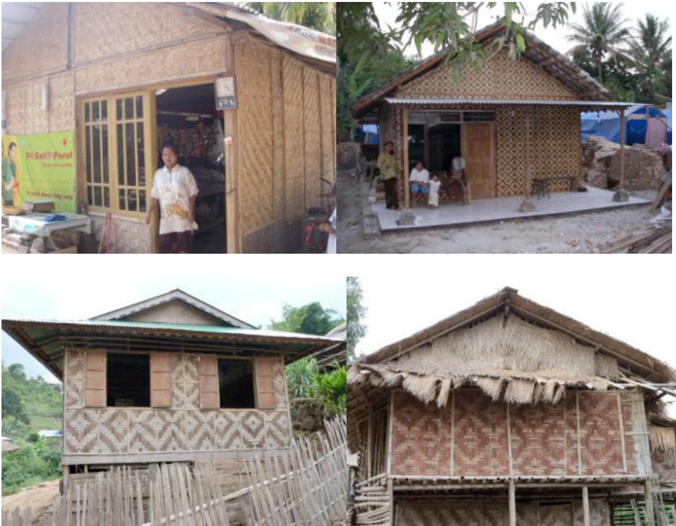
A RANGE OF BAMBOO CLADDING ON TEMPORARY SHELTERS
