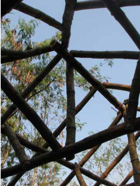
Step 2.G: diagonal braces from *bukpar* to tie-beams
