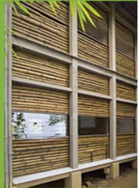
Probably the first and largest of its kind in India, Inspirations' office is built almost entirely with engineered bamboo – be it the floor and roof slabs and the walls. The office covering an area of about 2750 square feet was completed in Dec. 2002. It is noteworthy that almost 25% of the bamboo used in the building was obtained from the neighboring bamboo plantation. All the bamboo used for this building was treated with preservative treatment to meet functional requirement.
