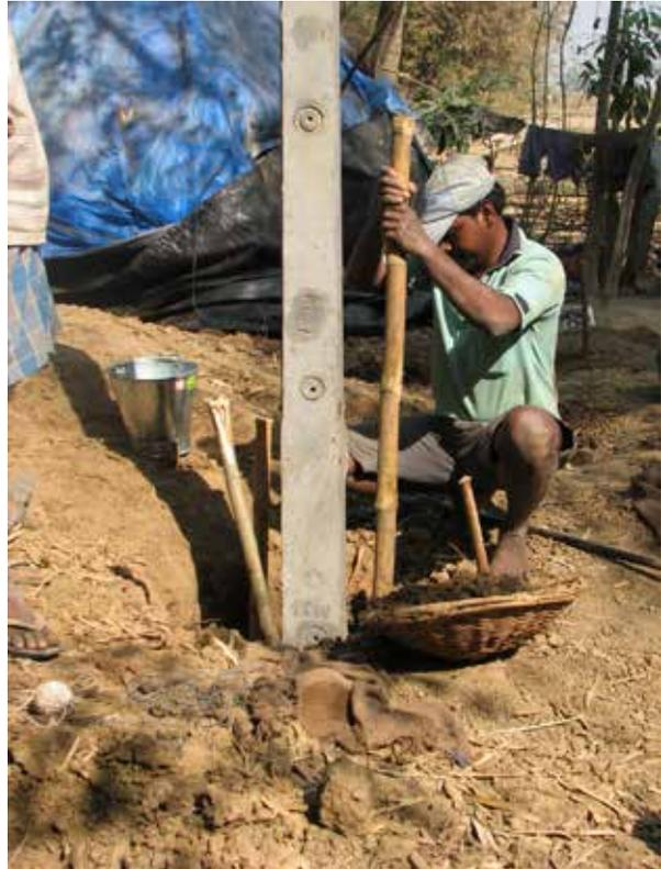
Step 2.C: pits filled and compacted
