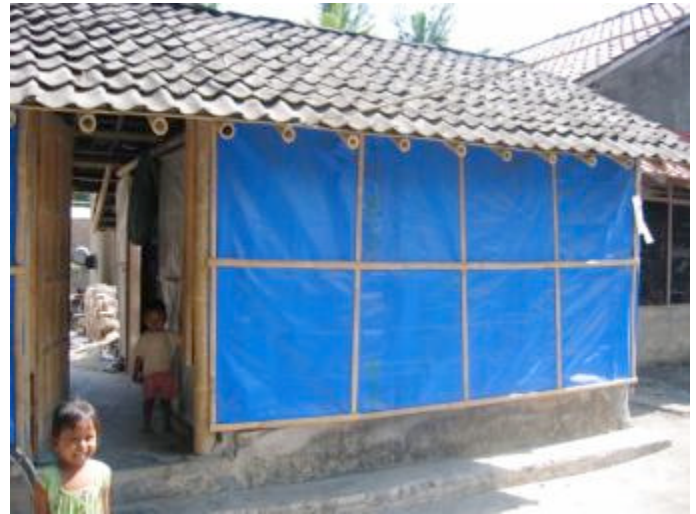
Plastic sheet walling on transitional shelter in Sewon, Indonesia
