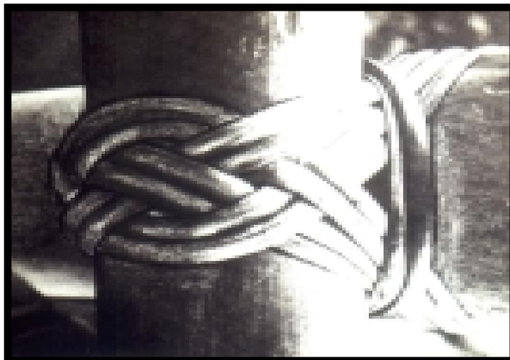
**Fig. 67:** Joint with rattan lashing (Dunkelberg 1985)
