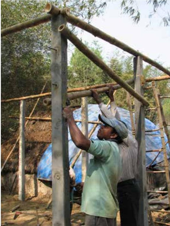
Step 2.D: cross-braces bolted at corner pillars
