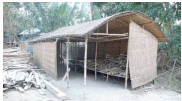
Temporary storage hut made from bamboo and jute
