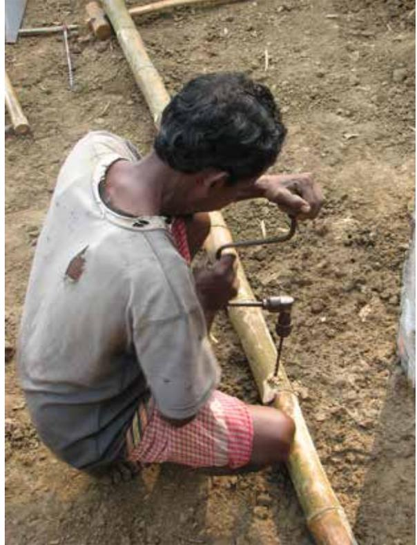
Step 2.D: top plates drilled and notched
