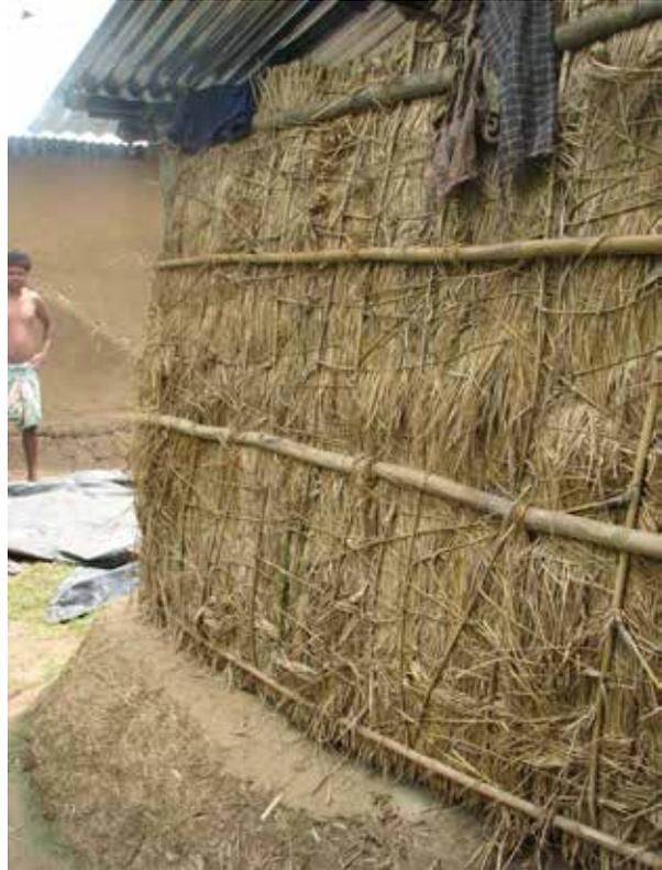
Step 5.A: exterior walls constructed
