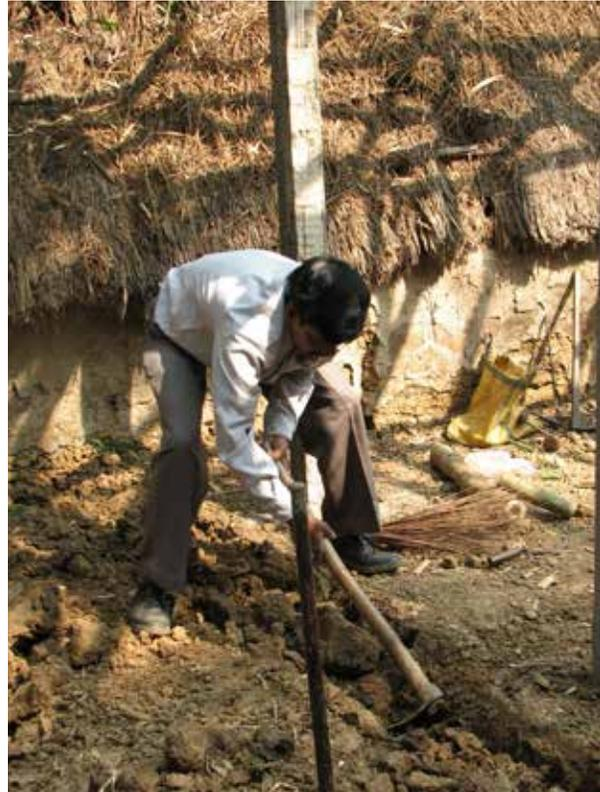
Step 3.E: drainage channels excavated
