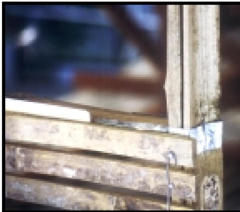
**Fig. 70:** *Joint for the upper corner of doorframes*
