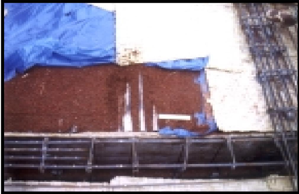
**Fig. 83:** *Woven bamboo mats in concrete formwork (Bangladesh)*
