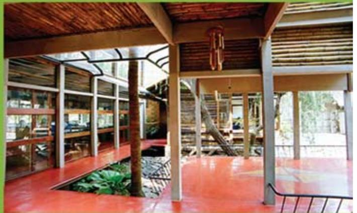
Bamboo is used as a composite along with optimized RCC members, ferro-cement and limited quantity of reinforced plaster, so as to arrive at an attractive, functional and cost effective technology. Large glazed windows are given along all inward looking walls which give ample protected lighting and ventilation.
