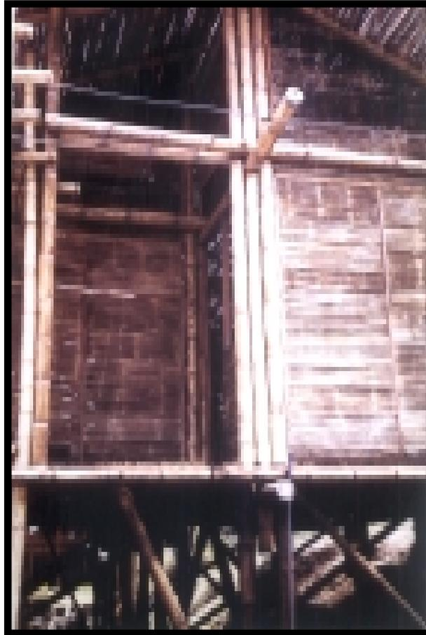
**Fig. 94:** A wall made of esterilla (Costa Rica)
