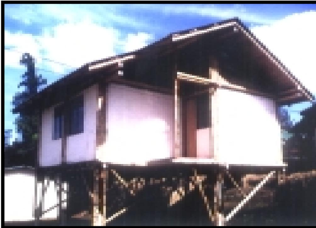
**Fig. 103:** *Prototype of a bamboo house with elevated floor (Costa Rica)*
