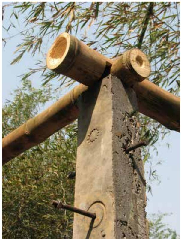
Step 2.D: top plates lapped and bolted at corners
