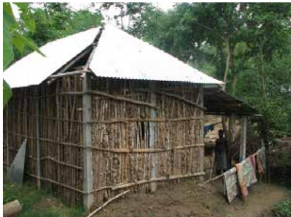
Step 4.A: CGI sheets cut to form four-sloped (hipped) roof
