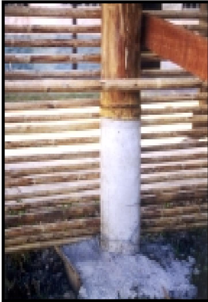
**Fig. 18:** *Prefab concrete foundation for bamboo column*
