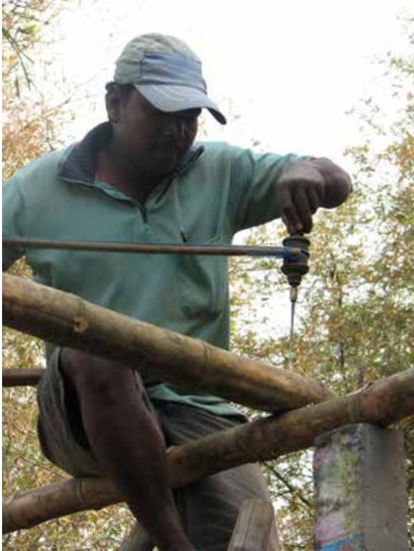
Step 2.E: tie beams pre-drilled and nailed
